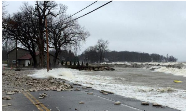
Figure 2: High water levels of a lake washing out a road [2].
